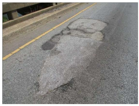
Span 10 Wearing Surface: (2) up to 9'-6" x 4' x 2" deep area of missing asphalt wearing surface with exposed rebar (PATCHED PRIOR TO 2022 INSPECTION)
