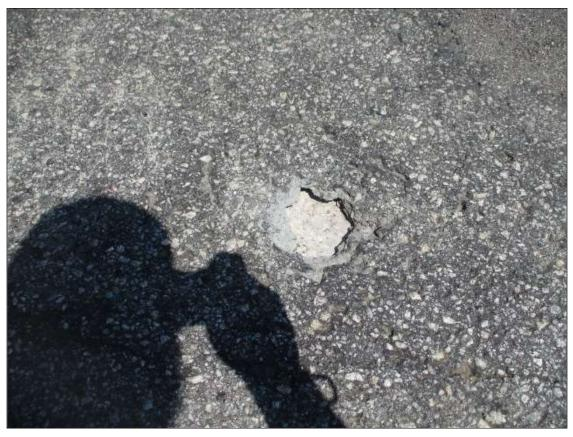
Span 10 Wearing Surface: (3) up to 8" x 6" x 1 1/2" deep area of missing asphalt wearing surface with exposed deck (PAR)
