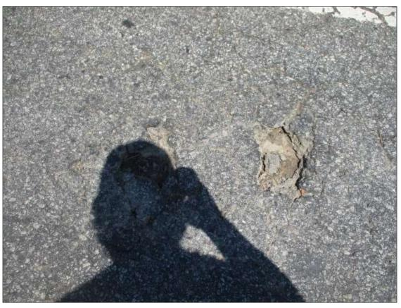
Span 8 Wearing Surface: [PAR] in both travel lanes, two [2] potholes in right travel lane near midspan: [12in diameter x up to 2in deep]; in left travel lane 20ft from bent 8 [1.5ft x 1ft x 2in deep] both exposing the top of deck
