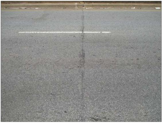
Span 3 Wearing Surface: asphalt over bent 2, multiple transverse cracks [up to full width x up to 1/4in]
