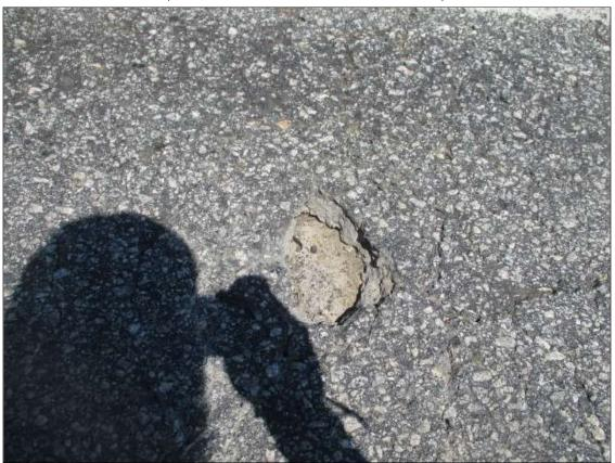
Span 10 Wearing Surface: (3) up to 8" x 6" x 1 1/2" deep area of missing asphalt wearing surface with exposed deck (PAR)
