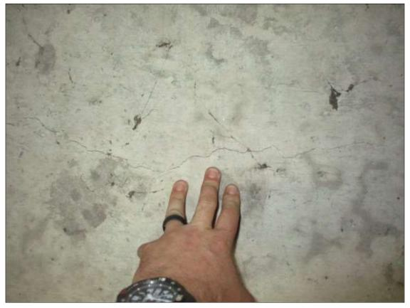
Bent 2 Abutment: 7' hairline horizontal cracks in Bay 1 (Bays 2 and 3 similar)
