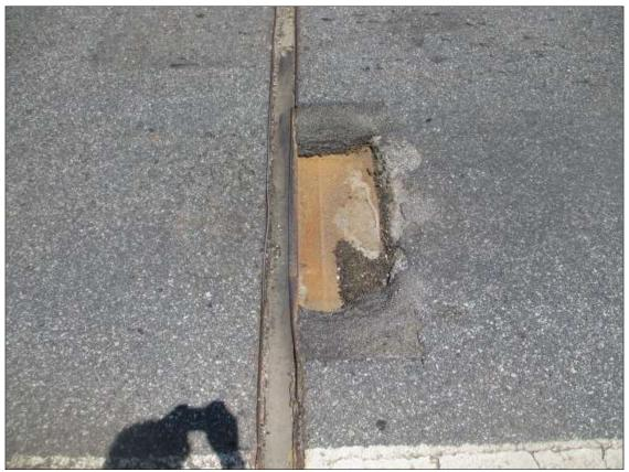
Span 10 Expansion Joint: (2) up to 14" x 12" x 2" deep area of missing asphalt wearing surface with exposed rebar along Bent 9 joint (PAR)
