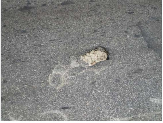
Span 1 Wearing Surface: PAR: 8" DIAMETER X 2" DEEP POTHOLE WITH EXPOSED TOP OF DECK IN LEFT LANE AT 15' FROM END BENT 1 AND 4' FROM WHITE LINE
