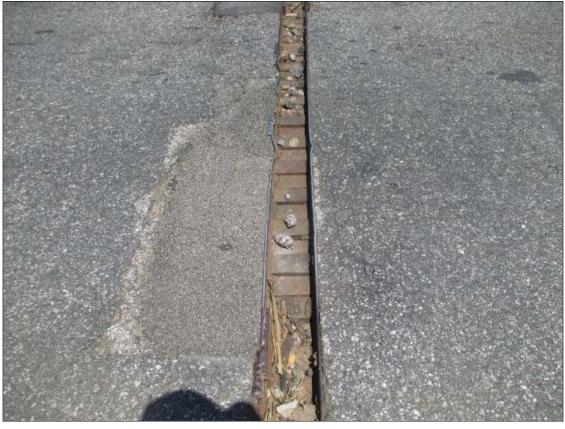
Span 2 Expansion Joint: [PAR] in right travel lane near dashed line, seal completely missing and adjacent metal angle distorted and sharp
