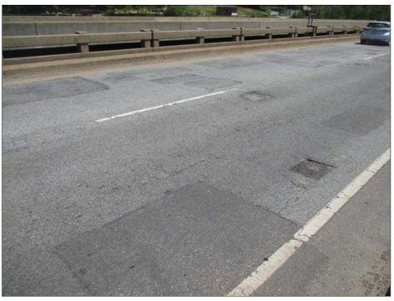
Span 9 Wearing Surface: throughout Span, (22) sound patches [up to 18ft x 9ft]
