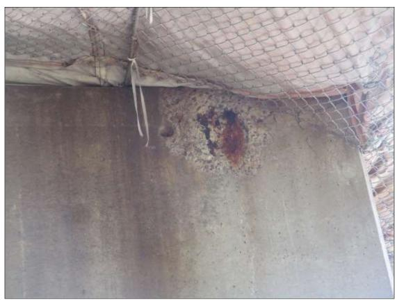
Bent 9 Cap 1: North face at West end, spall with exposed rebar and area of delamination [32in x 20in x 1- 3/4in deep] with two [2] exposed vertical rebar
