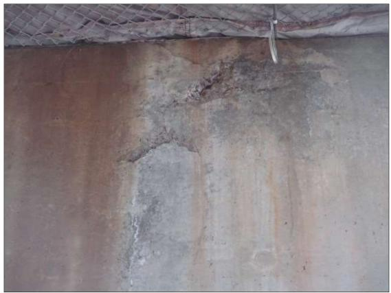
Bent 9 Cap 1: North face under beam 2, spall with exposed rebar and area of delamination [34in x 32in x 1-1/2in deep]
