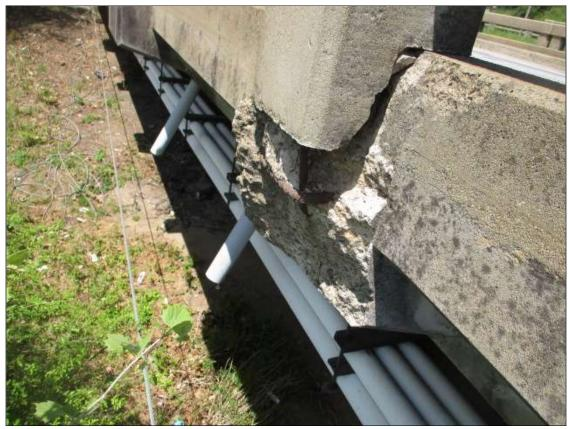
Span 10 Left Bridge Rail: 14" x 17" x 9" deep spall with exposed rebar on outside face of Post 5 (PAR)
