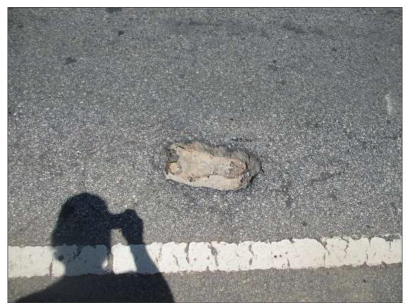
Span 7 Wearing Surface: PAR: 12" DIAMETER X 2" DEEP POTHOLE WITH EXPOSED TOP OF DECK IN LEFT LANE AT 10' FROM BENT 6 AND 1' FROM WHITE LINE
