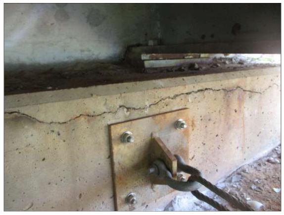
Bent 1 Cap 1: along length of cap below Bay 1, horizontal crack [up to 10ft x up to 1/16in] with 48" x 8" area of delamination
