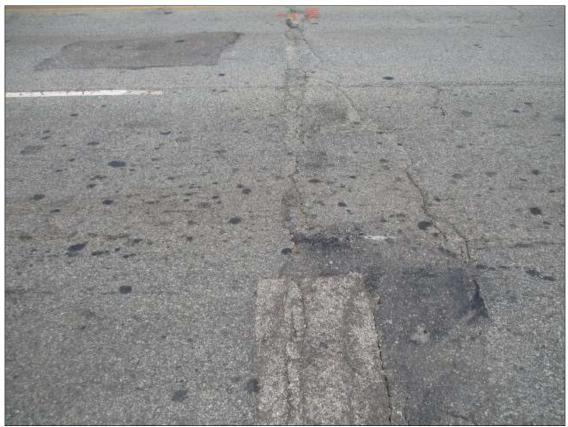
Span 1 Wearing Surface: asphalt over end bent 1 joint, alligator cracking [up to full width x up to 1/8in]
