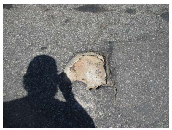
Span 8 Wearing Surface: PAR: 18" DIAMETER X 2" DEEP POTHOLE WITH EXPOSED DECK IN LEFT LANE AT 25' FROM BENT 7
