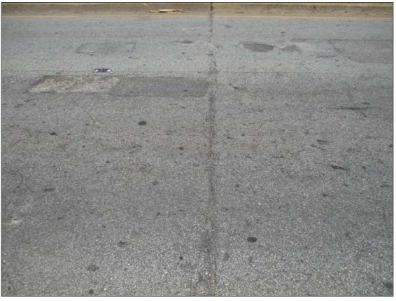
Span 8 Wearing Surface: 1/4" TRANSVERSE CRACKING OVER BENT 7
