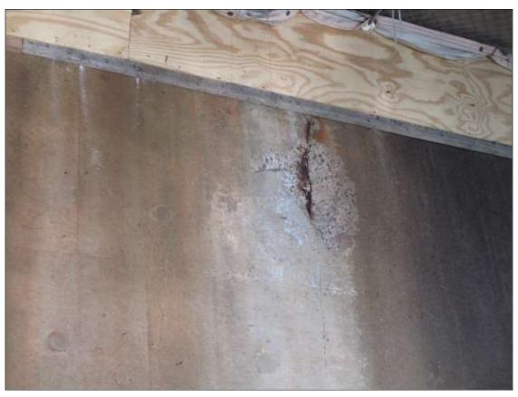
Bent 9 Cap 1: South face at beam 3, spall with exposed rebar [27in x 21in x up to 2in deep] with one [1] exposed vertical rebar
