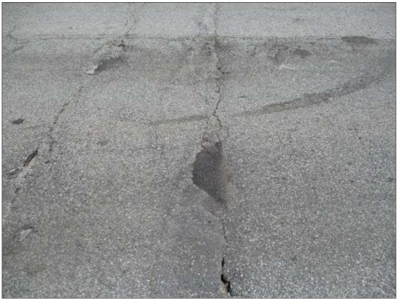
Span 10 Wearing Surface: asphalt over end bent 2, multiple transverse cracks [up to full width x up to 1/4in]
