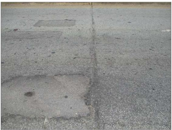
Span 7 Wearing Surface: asphalt over bent 6, multiple transverse cracks [up to full width x up to 1/4in]
