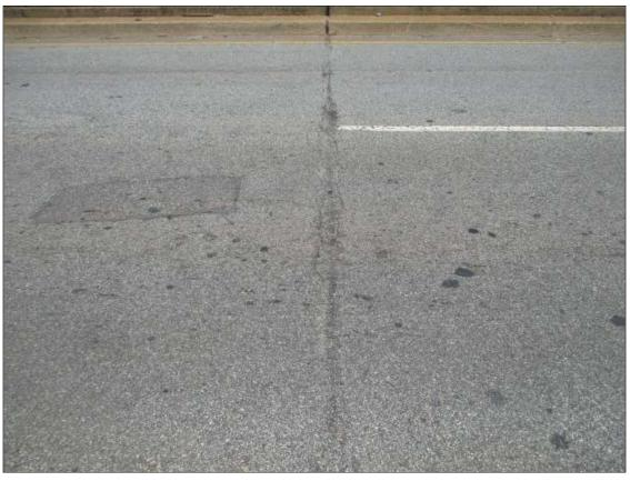
Span 5 Wearing Surface: asphalt over bent 4, multiple transverse cracks [up to full width x up to 1/4in]
