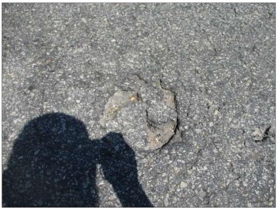
Span 9 Wearing Surface: [PAR] 13ft from bent 9 in West travel lane, pothole [8in diameter x 3in deep] exposing top of deck
