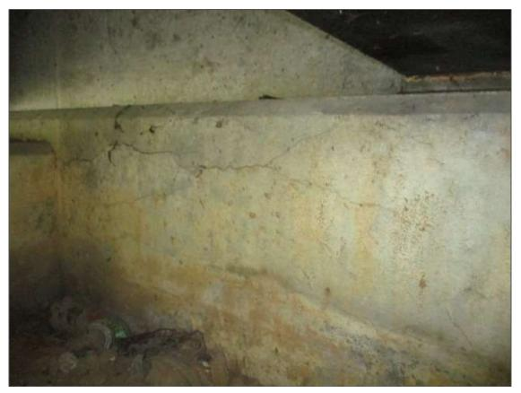
Bent 2 Cap 1: 11' up to 1/16" horizontal cracks under Bays 2 and 3
