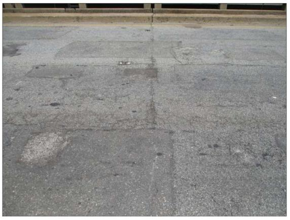
Span 9 Wearing Surface: 1/2" TRANSVERSE CRACKING OVER BENT 8
