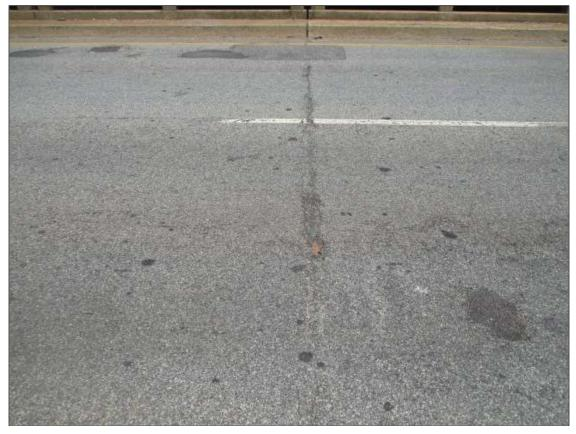
Span 4 Wearing Surface: asphalt over bent 3, multiple transverse cracks [up to full width x up to 1/4in]
