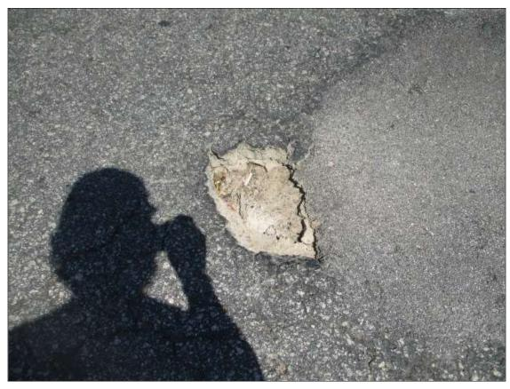
Span 7 Wearing Surface: [PAR] in LEFT travel lane, spall [9in x up to 9in x 2in deep] exposing the top of deck AT 6' FROM BENT 6 AND 2' FROM WHITE LINE
