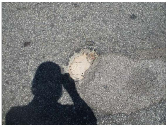
Span 6 Wearing Surface: PAR: 8" DIAMETER X 2" DEEP POTHOLE WITH EXPOSED TOP OF DECK IN LEFT LANE AT 15' FROM BENT 5 AND 2' FROM CENTERLINE
