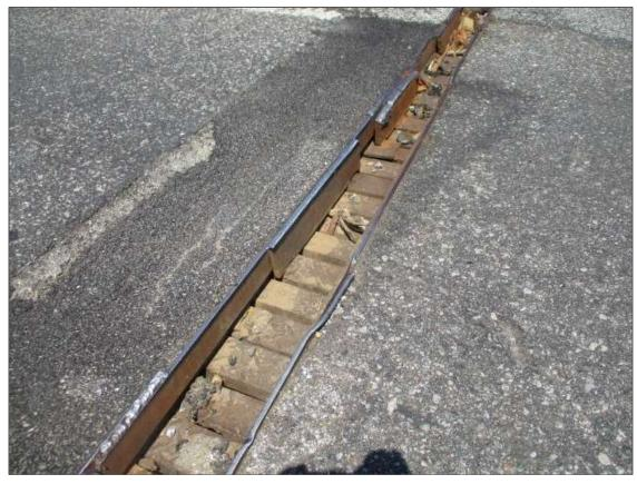
Span 2 Expansion Joint: [PAR] in right travel lane near dashed line, seal completely missing and adjacent metal angle distorted and sharp
