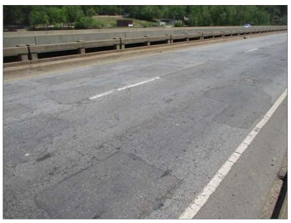
Span 8 Wearing Surface: (25) up to 15' x 4' area of sound patches
