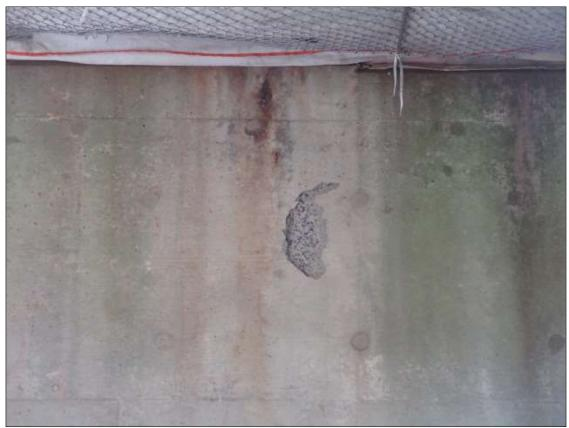
Bent 1 Cap 1: 22" x 33" x 1" deep spall and area of delamination on Span 1 face under Beam 3
