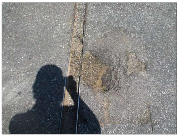
Span 10 Expansion Joint: (2) up to 14" x 12" x 2" deep area of missing asphalt wearing surface with exposed rebar along Bent 9 joint (PAR)
